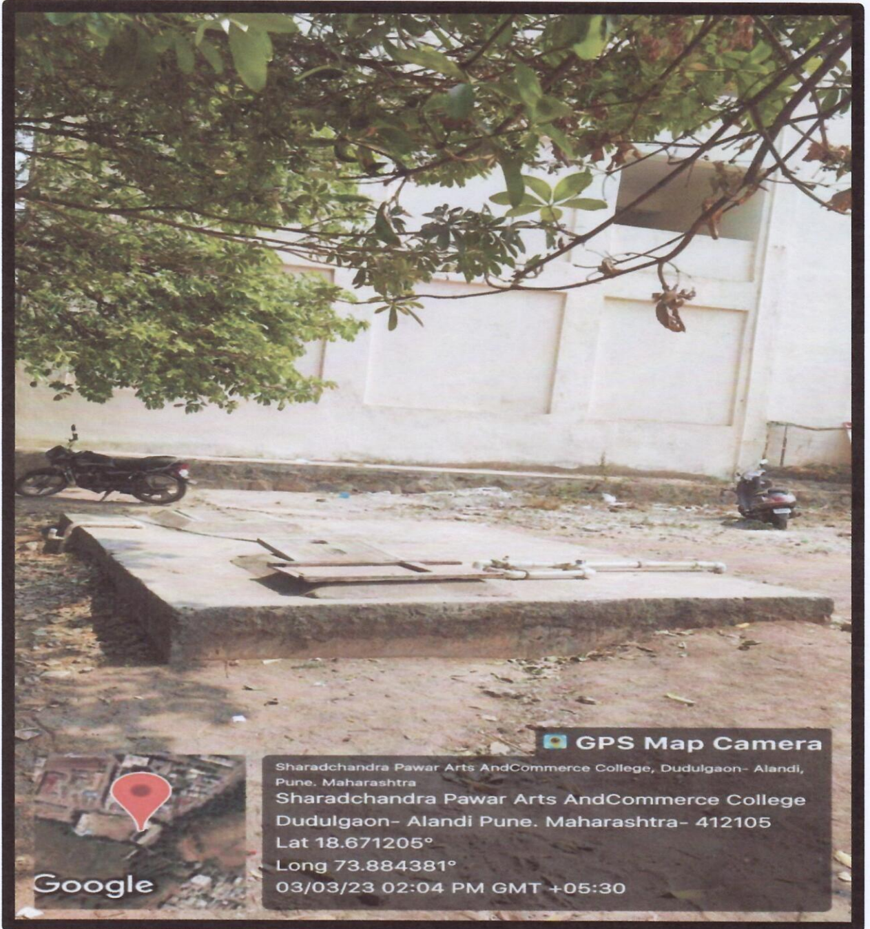
Ground Tank of Water
